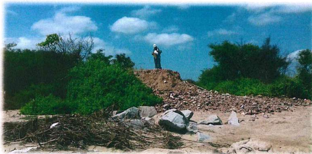
Foto N° 11, 12, 13: Dique Jayanca colapsado – Rio Motupe
