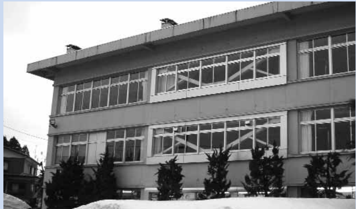
Façade of school after retrofitting
