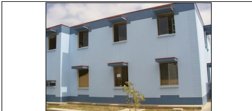
Figura 133. Hospital San Juan
