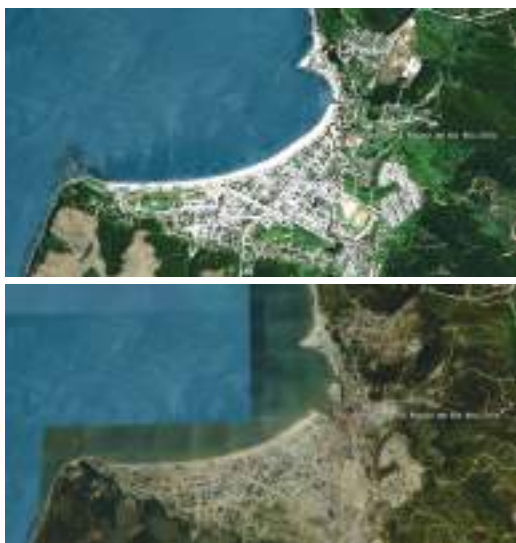
Figure 5.13: Before and after. Aerial photos of the damages caused by tsunami in Dichato
