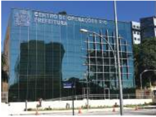
Photo 4.11: CO-RIO, City Government Operations Center
